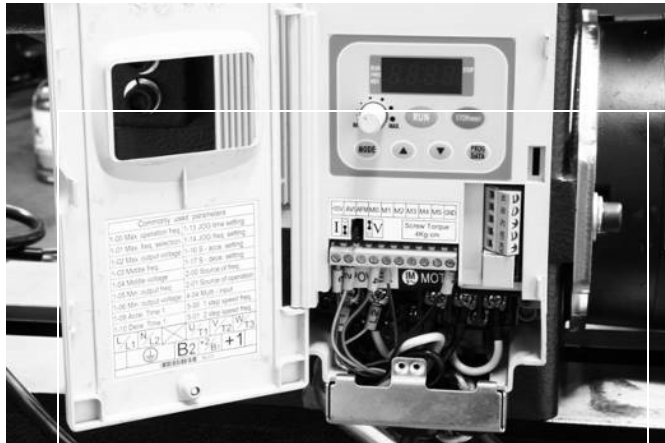
VFD with cover open
